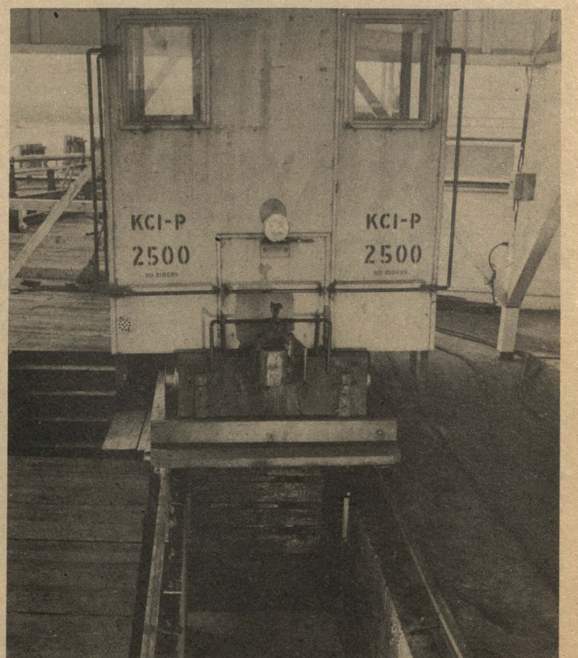
Repair Pit Inspection and repair of locomotives is made easy at this repair pit, located on the platform near the pump house. Previously, locomotives had to be lifted by cranes to blocks so Equipment Maintenance mechanics could get at working parts. Now the engine is run out on tracks over a sheltered pit. (Swan Island photo)
