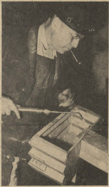
Walter Moore, Pipe Maintenance welder for 24 months, welds downspout which will go on Carpenter shop building. (Swan Island photos)
