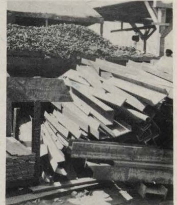
Scrap plate and angles are recut to specifications and returned to the ways. In background, part of a 60-day haul of bolts, nuts, washers.
