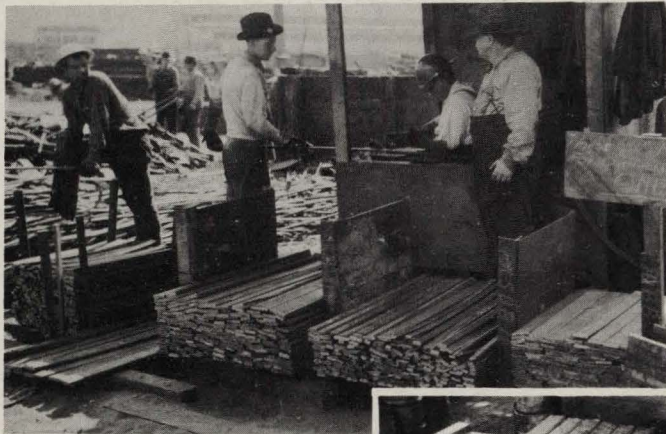
Strippings and scrap from plate shop are cut to size and returned to ways for use as inner-bottom stiffeners.
