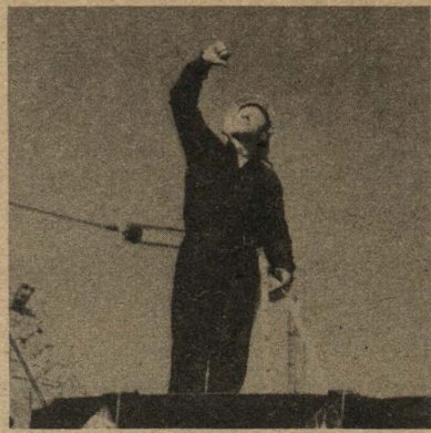
Boom Down Thumbs down doesn't mean the rigger has it in for the crane operator. Leadman Rigger D. S. Attebery wants the boom down.
