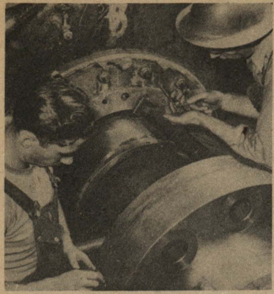
1. First operation for main propulsion motor crew is the alignment of tail shaft in stern tube. Leadman Hunt and Delplanche take the measurements.
