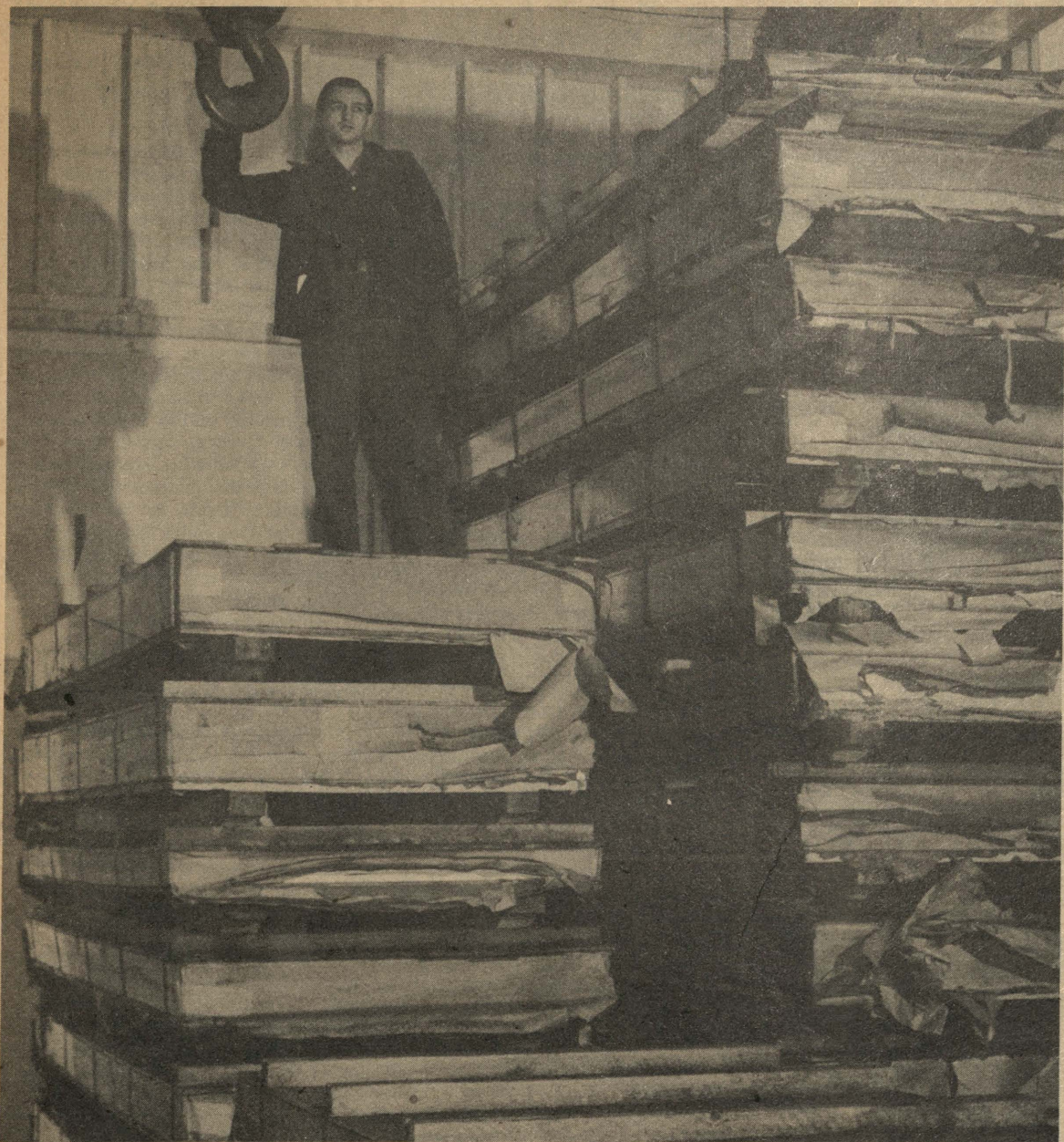
Ponton Plate J. H. Becker, OSC warehouseman, is pictured with part of the first shipment of aluminum plate to arrive in the yard for construction of 4000 half pontons for the army. Actual work on the pontons, which will play a major role in future invasions, will start during the first week in March. (Story, page 7)
