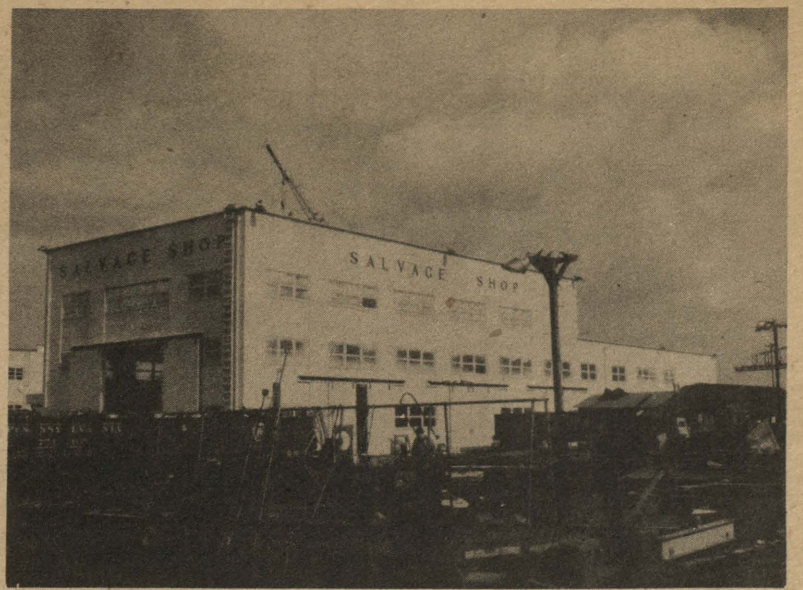
New Quarters Swan Island's new Salvage building was ready for occupancy last week when H. V. "Red" Sargeant's Labor department and J. A. "Archie" Sharar's Pipe Maintenance department moved in. The new building is located on the south side of the island across the tracks from Machinery storage. (Swan Island Photo)
