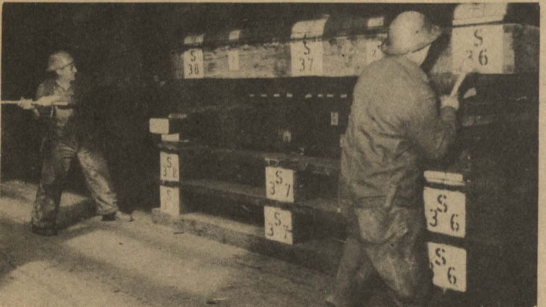
11:00 to 11:30 a.m. Tingum and Martin are removing bilge cribs prior to removal of dog shores (shown on front page) which takes place at 11:40. When dog shores are removed ship settles back with entire weight on burnoff plates. Standing ways slope 5/8-inch per foot and are cambered 3/4-inch per foot.
