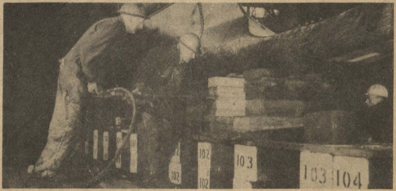
10:30 a.m. Under the stern Fred Michaels, M. Larson and Leadman H. Johnson use air driven chisel to split wedges. Johnson is using sledge. At the same time other workers knock loose shoring and keep blocks except bilge keel shores which later are ordered removed by Master Shipwright R. V. Sweitzer, who controls launching by telephone.
