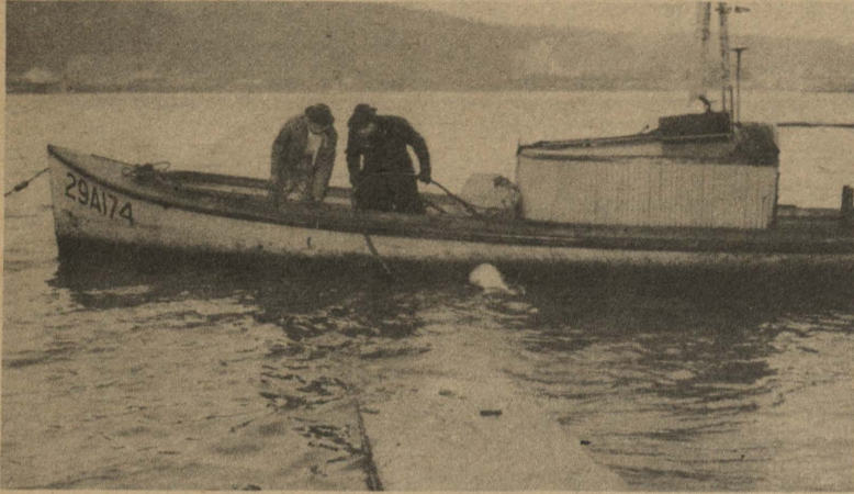
7:30 a.m. Diver "sweeps" ways prior to launching of SS Idaho Falls. For 1600 feet out and to a depth of 24 feet he explores the river bottom and at 9:30 a.m. reports condition of ways underwater. Divers are Devine and Zimmerman.
