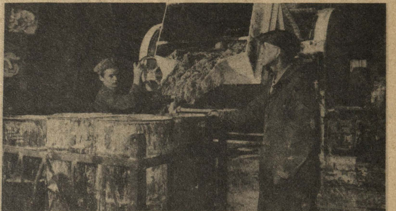
Bread Mixer An old bakery dough mixer is used here to mix "mud" for insulating tankers. Edwin Higham and R. E. McClelland dump a batch from mixer. (Swan Island photo)
