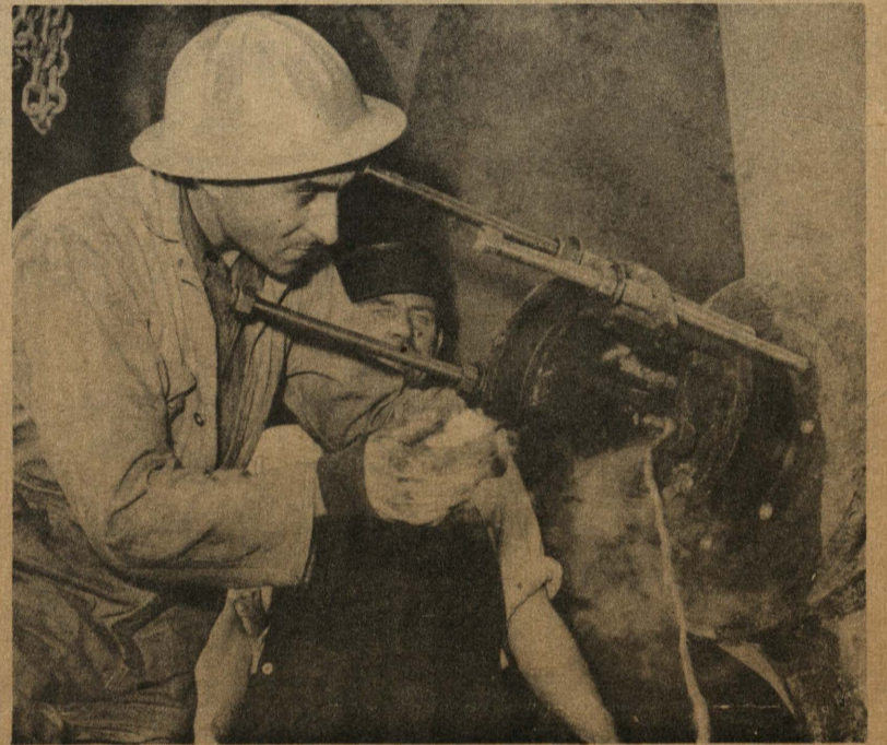
The Old Freezo On the Swan Island drydock, Farnam Johnson and Charles Crugaugh pack a hearing with dry ice to shrink it and allow the bearing to be pulled. Three feet long, the propeller shaft bearing has a taper of one-eighth inch. (Swan Island photo)
