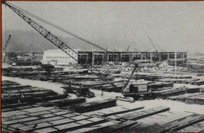
Part of the new Plate Storage Area at Oregon Shipbuilding Corporation. Over 1,000 tons of steel per day go from this area to the Plate Shop.
