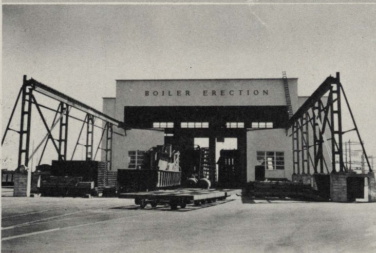
In this building the boilers for Swan Island's oil tankers are prefabricated.
