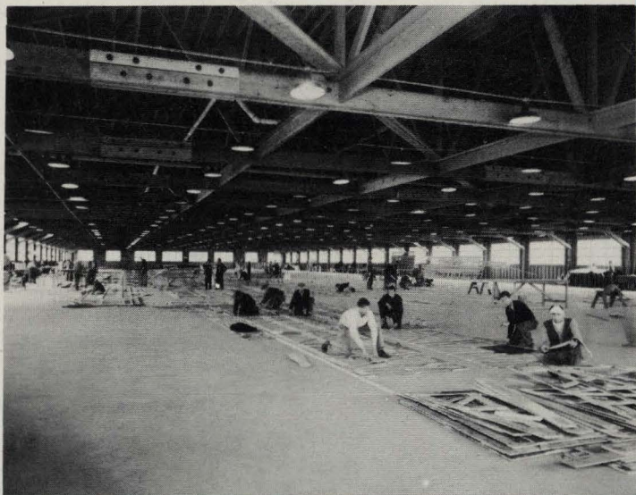
On this big Mold Loft floor, loftsmen make templates and patterns for tanker plates and sections.
