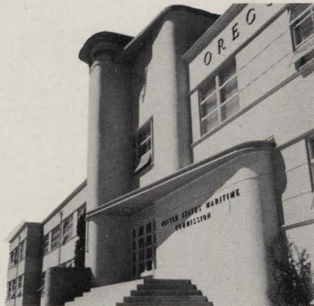
O. S. C. Administration Building
