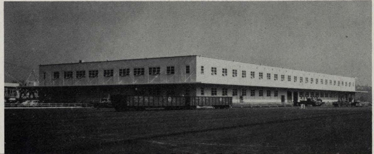
Another view of the General Stores building, with ample dock space for loading and unloading materials.
