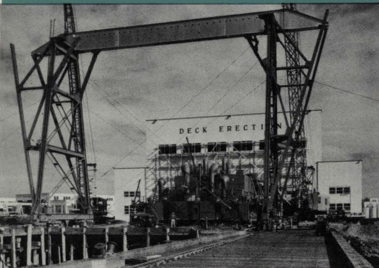
Ready to be lifted onto a ship is this 230-ton, three-story deck house. 215
