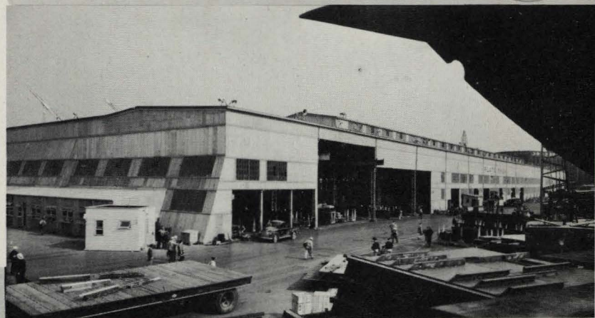
At the head of each ship way prefabricated sections are stacked, carried by cranes into hulls as construction progresses.
