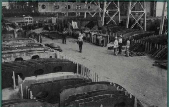
From the Plate Shop to the Storage Area at the Assembly Building come shapes stored in duplicate quantities—enough for 6 or 8 ships awaiting their place in the Assembly Building production line.
