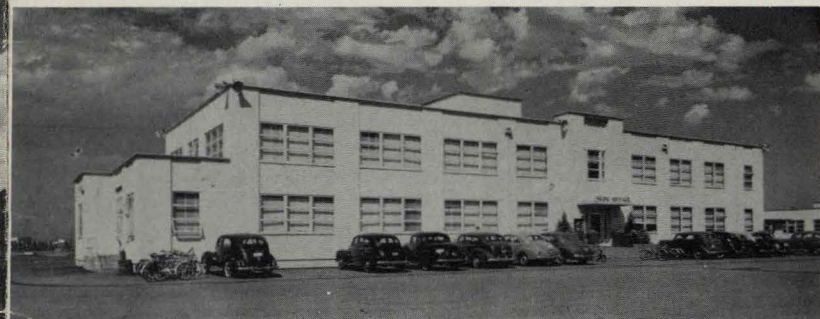
The Vancouver yard office, where construction detail and administration are handled.
