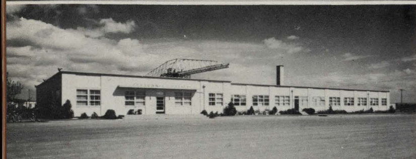
Near the Vancouver Administration Building is this separate personnel office, where War Bonds, Insurance, and other personnel matters are handled.
