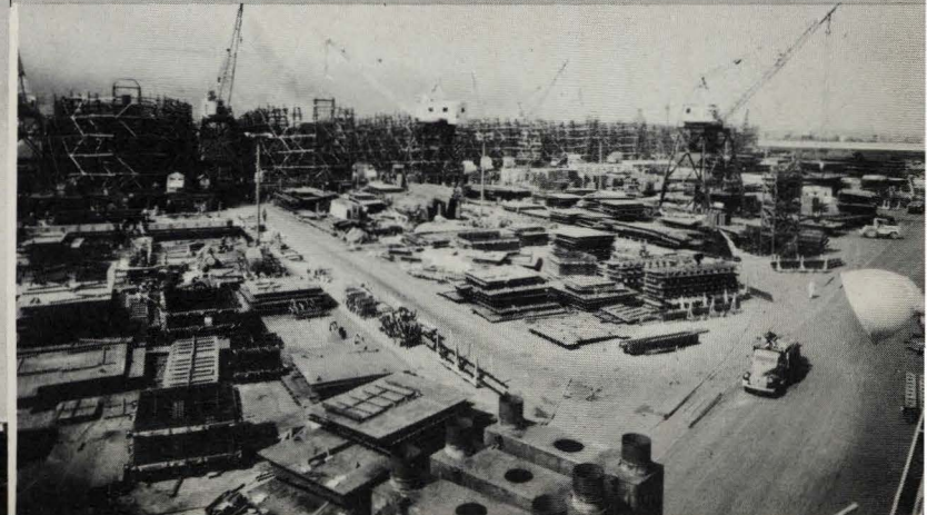
At the head of each ship way prefabricated sections are stacked, carried by cranes into hulls as construction progresses.
