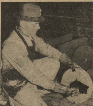
John A. Bennett, painter at the Buckler-Chapman Joiner plant, applies a coat of "Victory ship grey" to a wooden instrument base. Besides instrument bases of assorted sizes, the plant turns out hardwood bases for laundry room and galley equipment for BB3's, and telegraph, drill press and steering stand bases for both BB3's and Victory ships.
