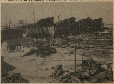
Not too much unlike present yards is this view of the ways. Note the "cranes" at each way. The yard built wooden and steel ships.
