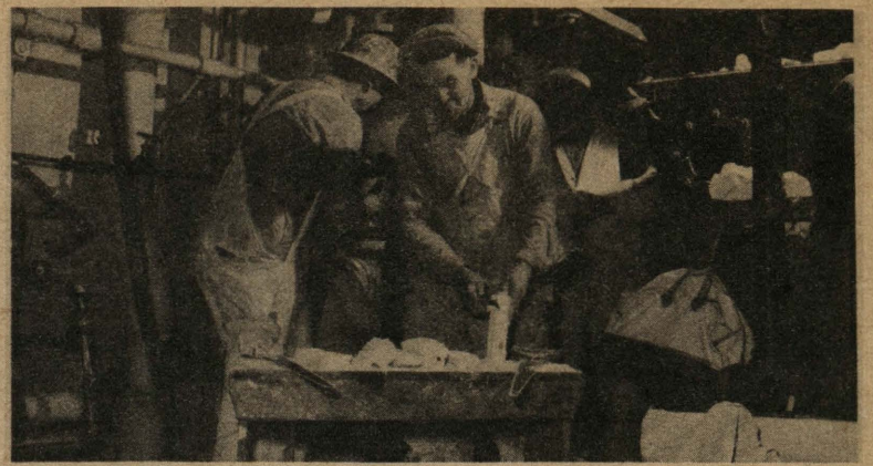
Asbestos Men Charles Snyder, Phil Smith and Hy Pi-fer fit asbestos insulation on boiler room pipes of a Swan Island tanker at the Outfitting dock. (Swan Island photo)
