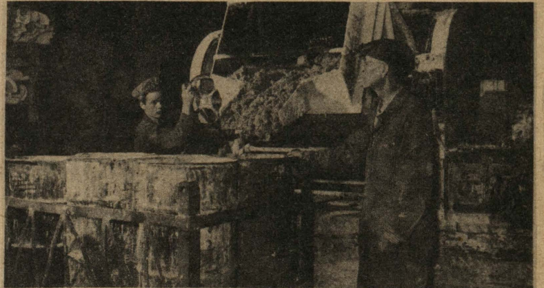
Bread Mixer An old bakery dough mixer is used here to mix "mud" for insulating tankers. Edwin Higham and R. E. McClelland dump a batch from mixer. (Swan Island photo)
