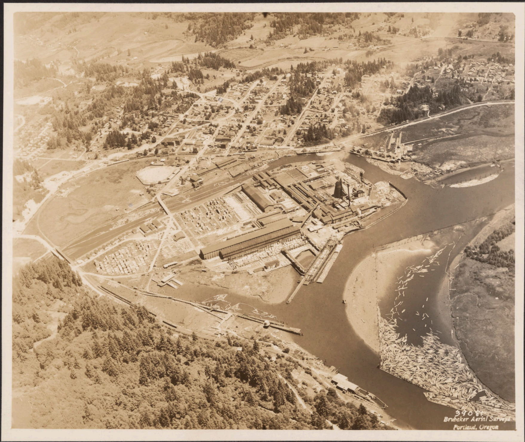
TOLEDO AND C. D. JOHNSON MILL IN FOREGROUND
