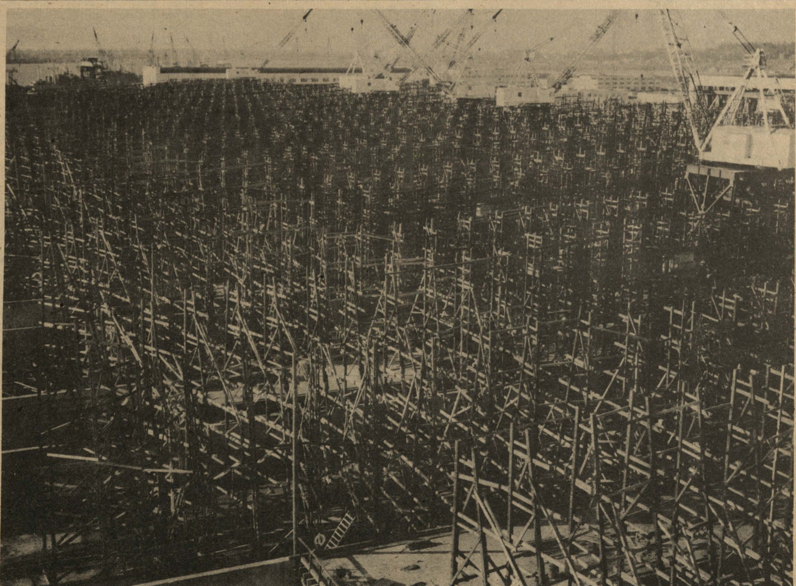
C-4's A 'Bornin' The ways, shown above before Christmas when they appeared like a great forest, are now beginning to show visible signs of great ships' hulls again. Hull 501 is half erected, according to latest Progress department reports, and Hull 502 is coming along on schedule. (Vancouver photo)
