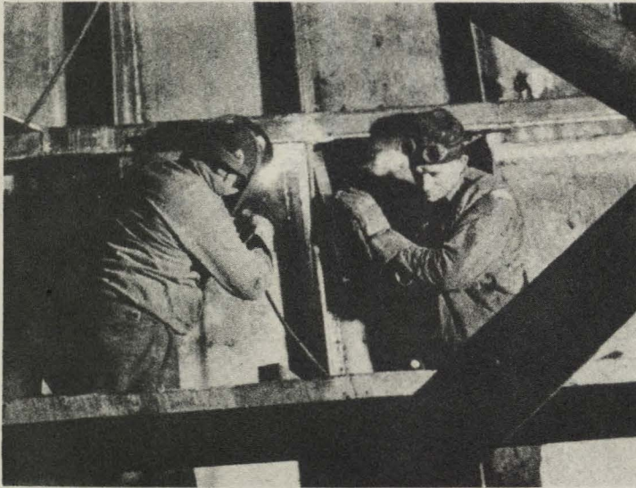
Rivetless ship having its ribs securely welded to the hull plates. Saving in weight, great strength, and rapid fabrication results.
