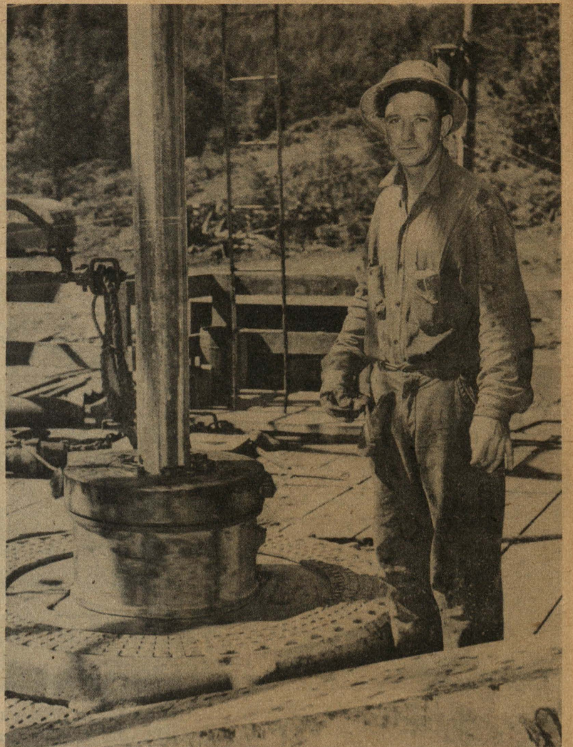
Drilling The disc-like installation on the rig floor is a rotary table, which imparts the rotary motion to the drill pipe and the bit through the hexagonal Kelly that extends from the rotary table to the top of the picture. The workman is a pipe-racker.
