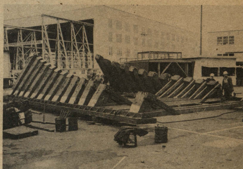
Mastodon Like the skeletal ribs of some prehistoric mastodon being unearthed in the desert are the timbers of this section of the sliding ways. (Swan Island photo)
