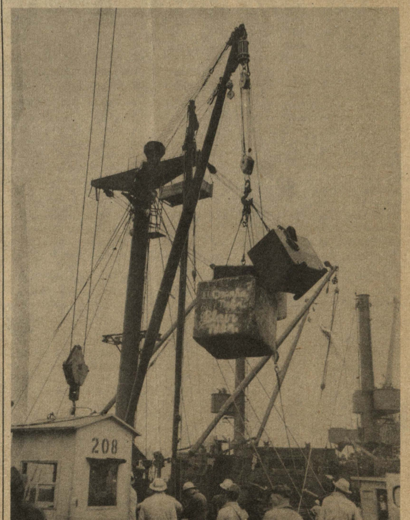
Boom Testing Sixty tons of concrete and steel are lifted by the boom on this navy ship at the Swan Island Repair dock. This is three times as much weight as the booms ever are expected to handle.
