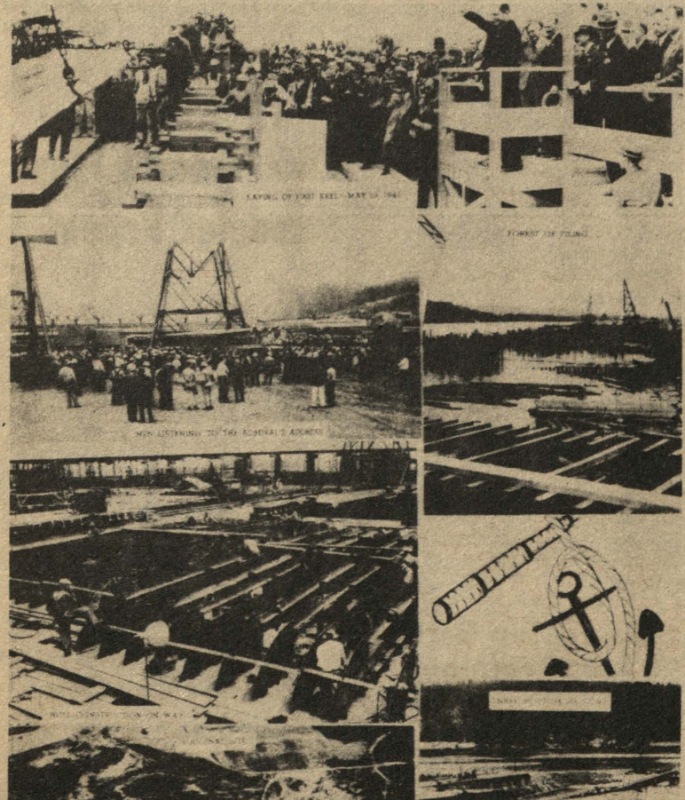
Oregon Ship workers thought their yard had gone quite a ways in the first six months of its existence, and the first edition of the Bosn's Whistle, issued as a small magazine on July 18, 1941, printed a page of pictures to illustrate progress made. The photographs show the Star of Oregon keel-laying, double bottom fabrication, hull construction on ways, the yard's original site, and piling.
