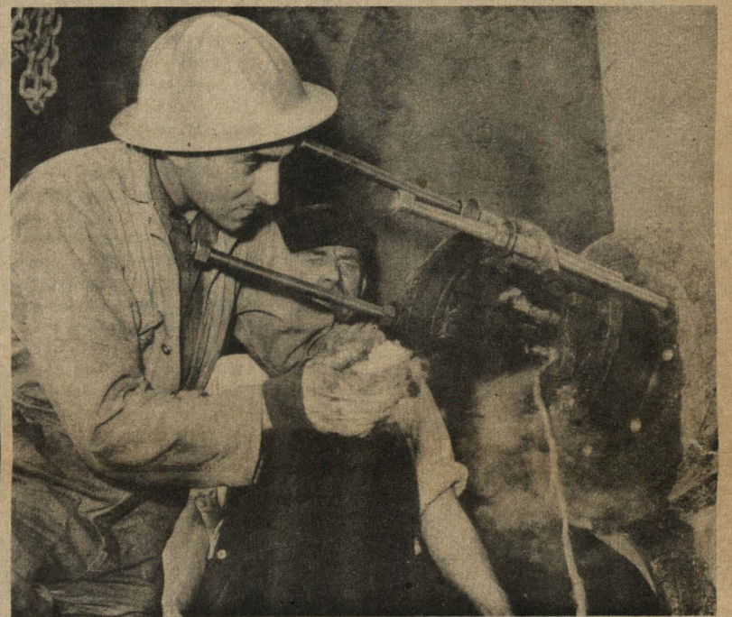
The Old Freezo On the Swan Island drydock, Farnam Johnson and Charles Crugaugh pack a hearing with dry ice to shrink it and allow the bearing to be pulled. Three feet long, the propellor shaft bearing has a taper of one-eighth inch. (Swan Island photo)
