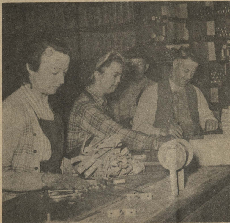
In the lay-out assembly shop, cable hangers, raceways and kick pipes are pre-assembled to be sent to ship in kit form ready for installation. The four above are part of day shift crew. They are, left to right: Margaret Baker, Juanita Sharp, A. L. Freeze and E. L. Reneau.
