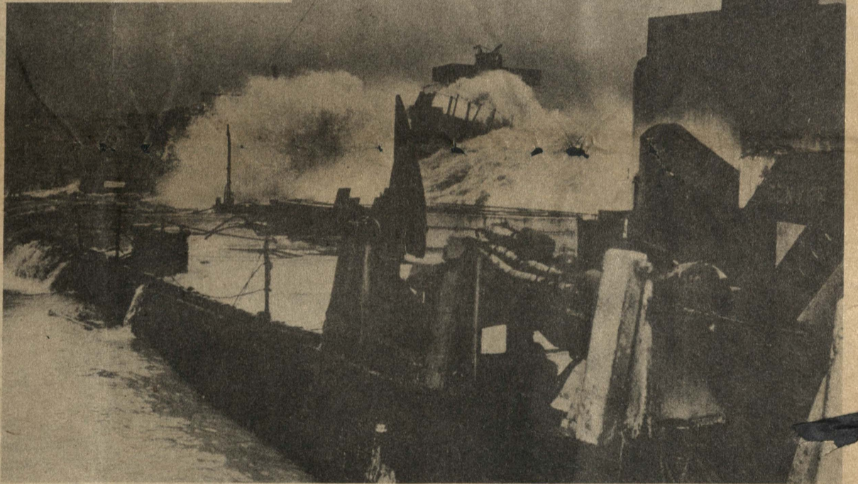
Improved Harbor Heavy seas, threatening to demoralize the Normandy landings soon after D-Day, beat against a barricade of sunken ships a half-mile off shore. In a carefully planned operation carried through in the wake of the landings 23 ships including Libertys and old tankers, were loaded with cement and "scuttled" to form an improvised breakwater behind which landing craft were unloaded. Above, a mountainous wave spends its fury against the Centurion, key ship of the chain. Below, this is how the breakwater looked before the storm hit. (Official U.S. Navy photo)
