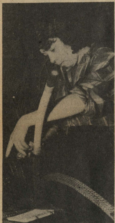
Mildred Stevenson prepares cable-ends. There are 35 of this type cable for each ship. Cables are stripped, harnessed, wrapped, varnished and cut to proper size for installation.
