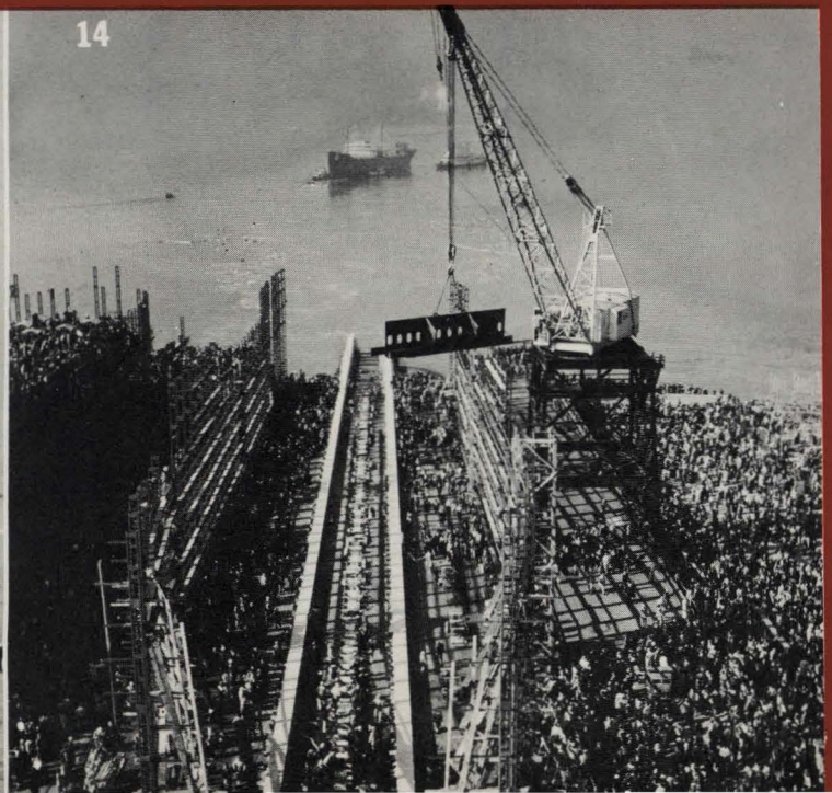
14 They're not fooling at Swan Island. With the "Schenectady" still in the river, new keel plates swing into place.
