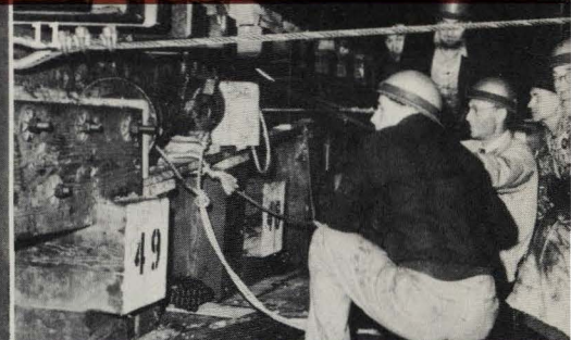
12 "Burn-off" plates holding the tanker have 13 holes — broke after the 11th had been burned. Here a burner is cutting thru the first.
