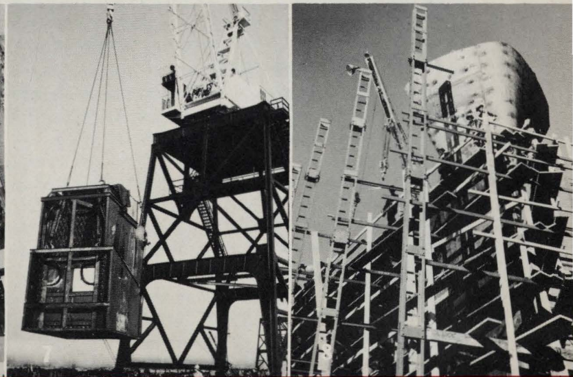
7 Giant boiler weighing 52 tons when erected is hoisted on board.
