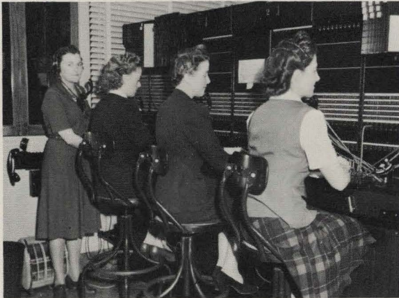
Oregon switchboard artists. In the foreground, Mrs. Cora Lee Newell, chief operator. At board, left to right, Virginia McNair, Maude Anderson, Ida Salyer, Bessie Brink, Effie Wilson
