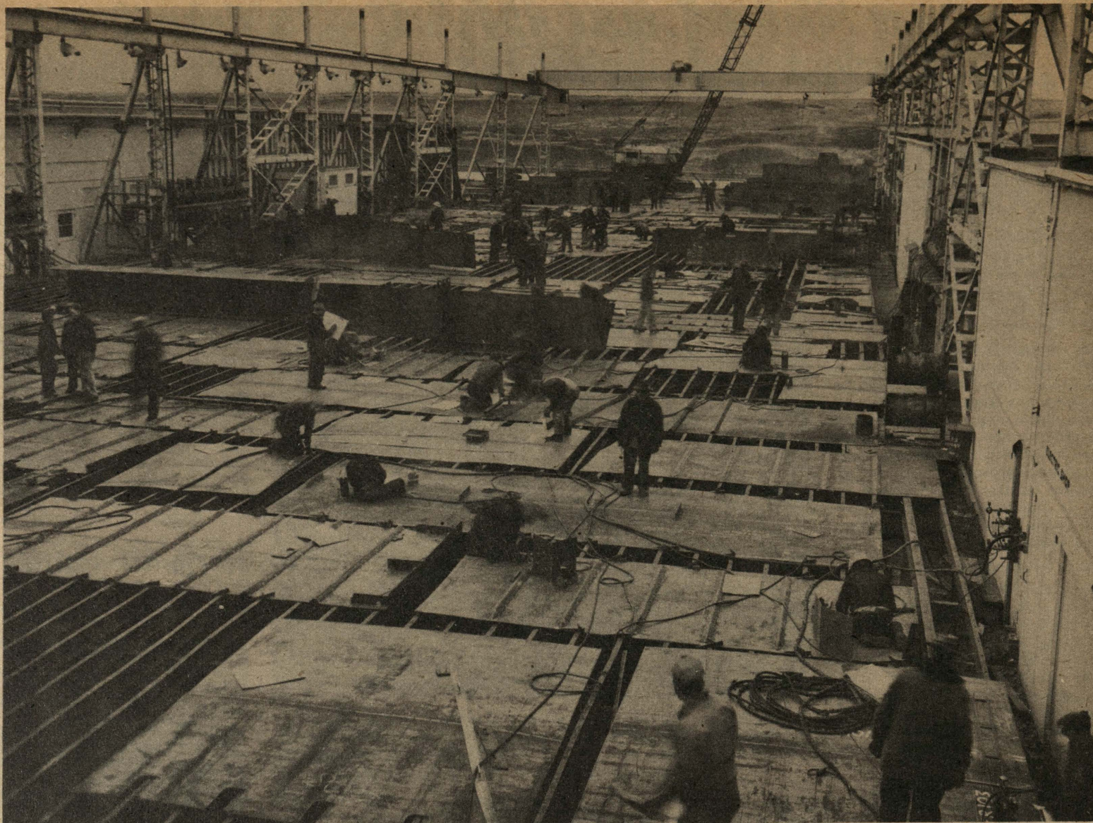
KCIV--The Dalles Looking north from the assembly plant at The Dalles, Oregon, toward the Washington side of the Columbia river provides this over-all view of the key up-river plant of the Vancouver yard. Work done here is shipped by barge to Vancouver.
