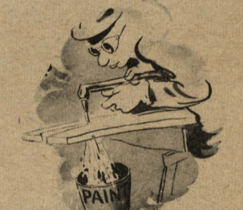
Paint should be covered; should not even be in the vicinity of the burner's torch. But it happens!
