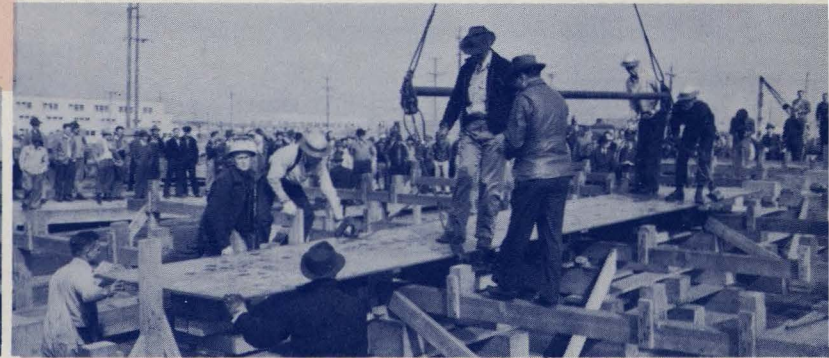
Laying the first Liberty Ship keel at Vancouver on April 15.
