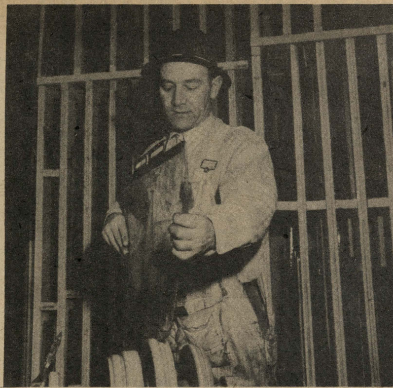
Standing in front of racks filled with glass for Oregon Ship's future broken windows, Joe Miller, yard glazier, grinds rough edges from a truck windshield. Miller repairs any broken windows and glass gadgets used in the yard.
