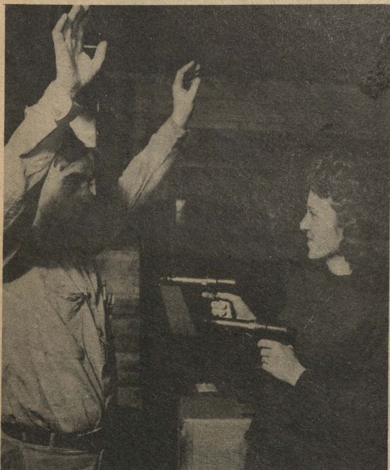
Stick 'Em Up! It looks like a holdup, all right, but there is nothing lethal about the two "weapons" that Mary Helen May, OSC warehouse clerk, is pointing at Leadman R. L. (Shorty) O'Dell. They are rivet guns which will be used in construction of 4000 aluminum pontoons for the army. A shipment of 310 of the guns arrived at the warehouse last week. (Oregon Ship photo)
