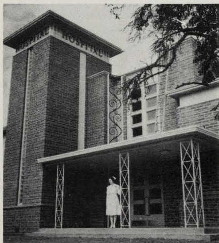
Main entrance and central tower of the 350-foot long building. This tower faces the majestic Columbia River and almost every room has a view of the river and the mountains. Nurses' station, which has direct speaker connection with each room and ward, as well as flash system. Corridors are unusually wide for speedy and efficient service.
