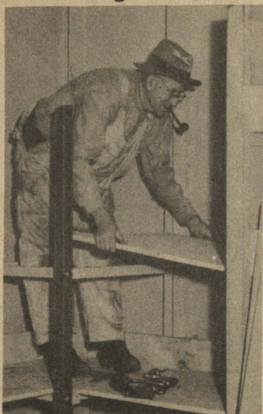
O. B. "Bill" Dillinham, O.S.C. Buckler-Chapman joiner, puts in a section of shelving in a dry storage space, for canned goods storage.
