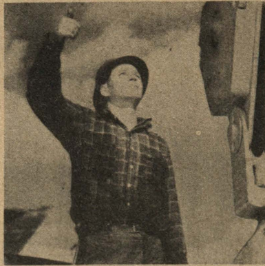
Boom Up Rigger Marvin Bragee, Vancouver, isn't trying to hitch a ride to heaven. He's signalling the crane operator to raise the boom.
