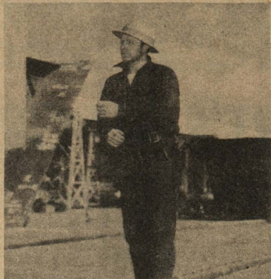
Travel Rotating his hands and arms, Leadman Rigger D. S. Attebery of Vancouver signals the crane operator to keep moving, a part of riggers' sign language.
